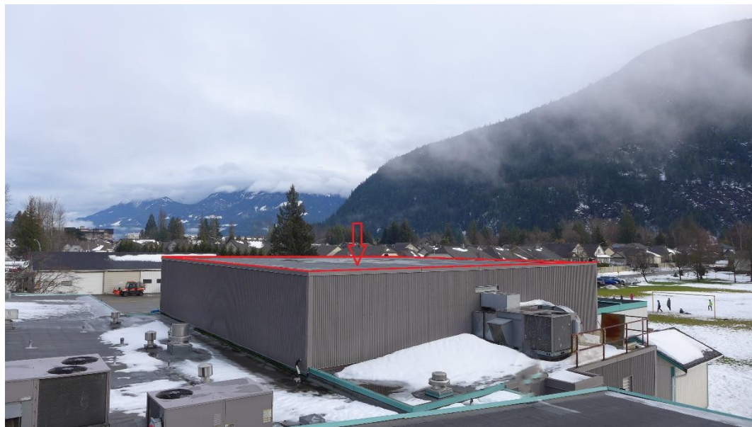
Figure 3: Site for Rooftop Solar Installation
